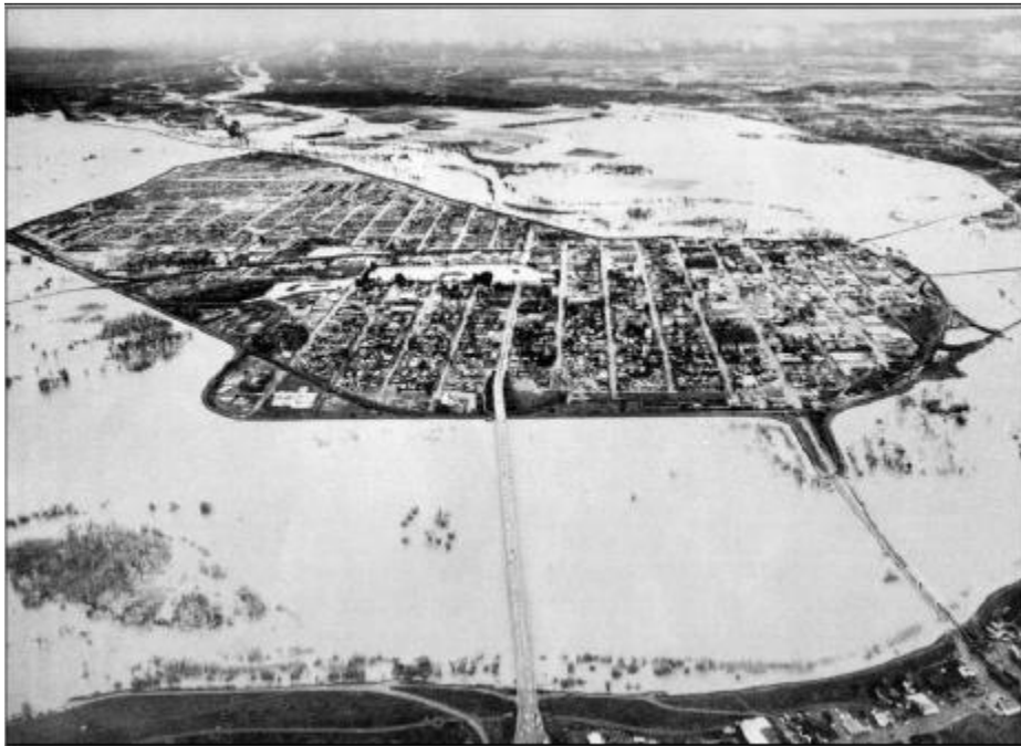
Figure A-18 City of Marysville – 1955 Flood Surrounding the City
